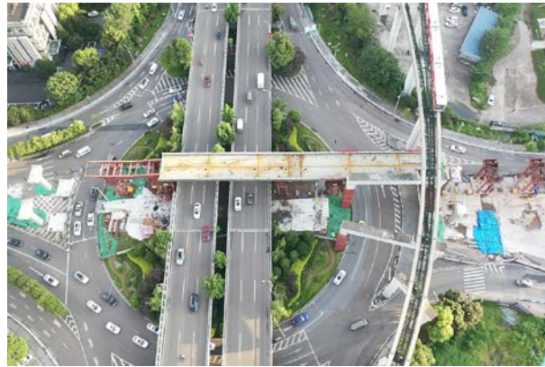
Fig.5 Construction Site of Steel Box Girder Top Push
